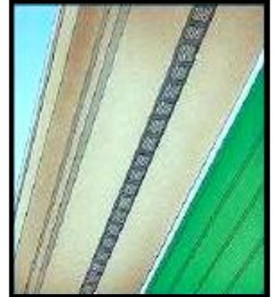
**Continuous Soffit Vent**
